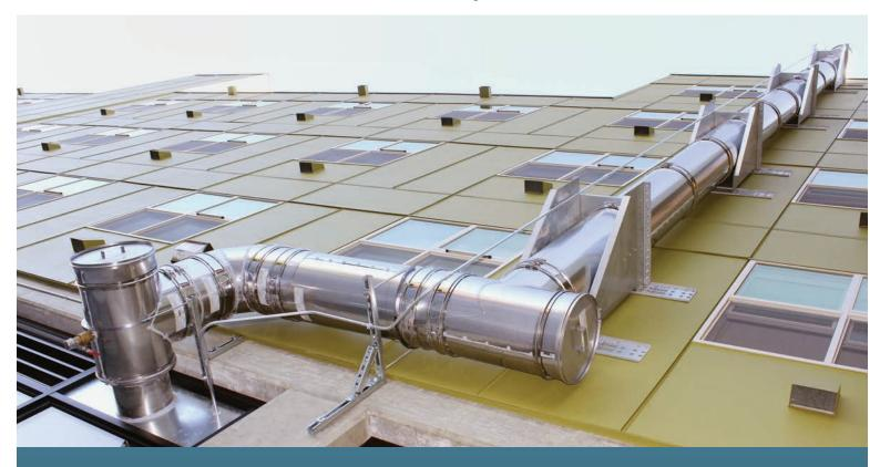
DOUBLE WALL GREASE DUCT
